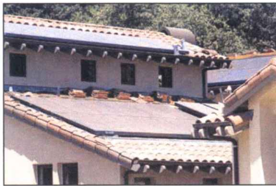
Two 4-by-10-foot solar panels on the roof instantly convert sunlight into electric power; if the homeowner is on vacation, the PG&E meter actually spins backwards.
